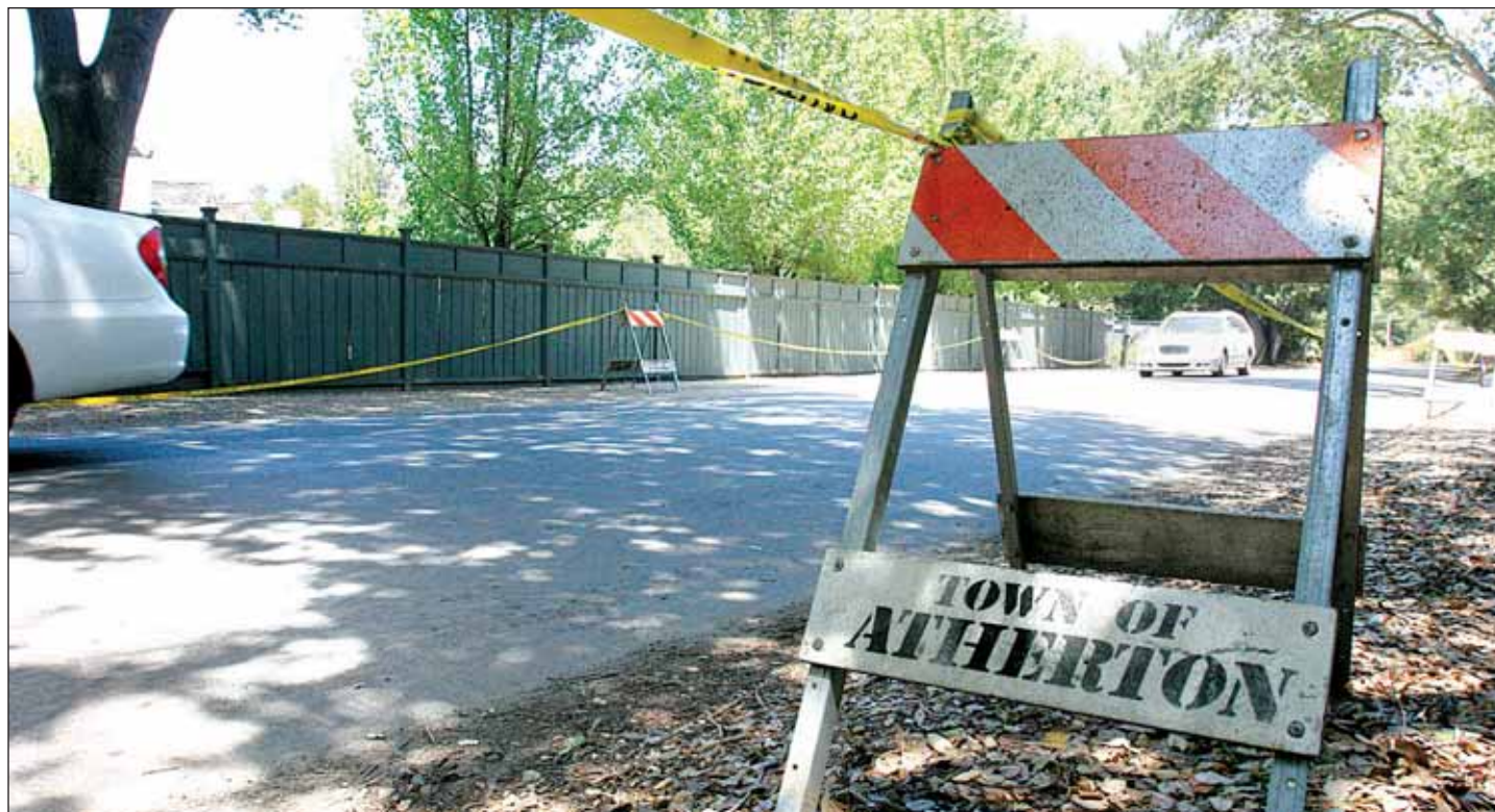
The Almanac/Marjan Sadoughi Construction sign on Park Lane in Atherton. A recent count showed that Atherton had about 110 residential construction projects going on in a town
