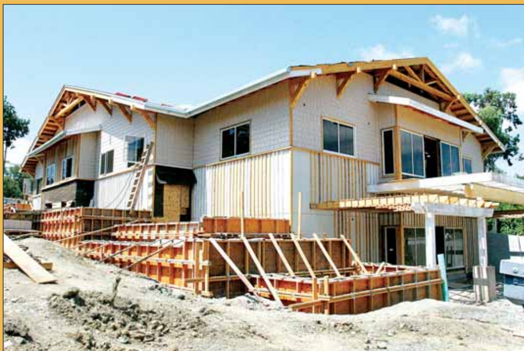
Woodside fire's new station is nearing completion.
