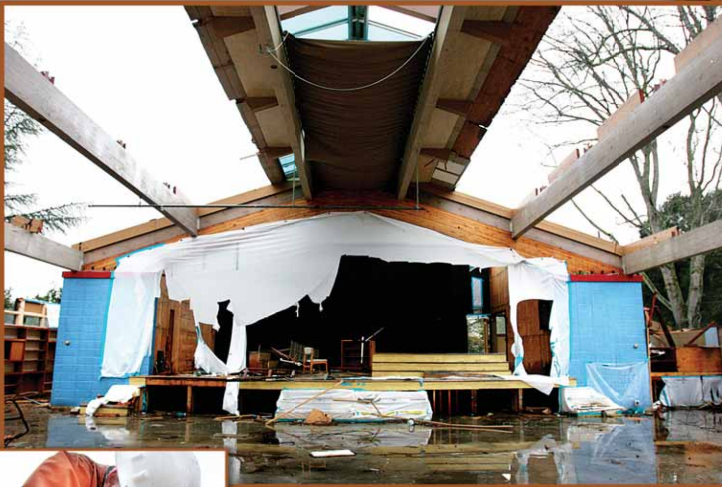
Above: The rafters once spanning these gaps in the roof of the multi-use room at Portola Valley Town Center will have a second and more visible career in the interiors of a new Town Hall, library and community hall. Left: Jim Steinmetz tightens the band around a stack of tongue-and-groove boards from the roof of the former Portola Valley School. Mr. Steinmetz led the dismantling of the school buildings.
