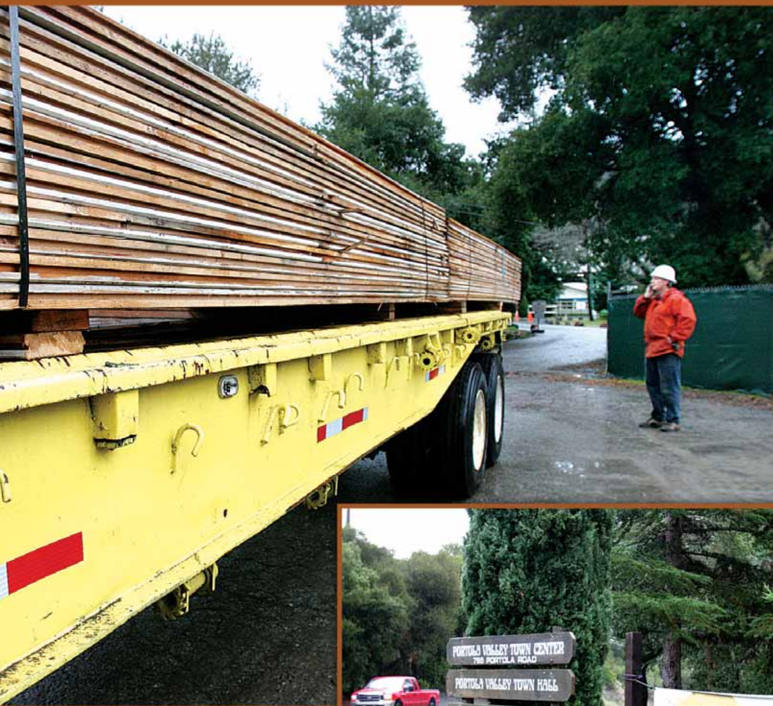
Left: Reusing this wood in the new Town Center complex lowers by 90 percent the environmental impacts of lumber transportation. Woodside resident Jim Steinmetz, owner of the Reusable Lumber Co., organized the recovery, transport and re-milling of 14,000 linear feet of lumber from the former Portola Valley School. Below: A recycling notice may be up until late in 2008 as Portola Valley rebuilds its Town Center.
