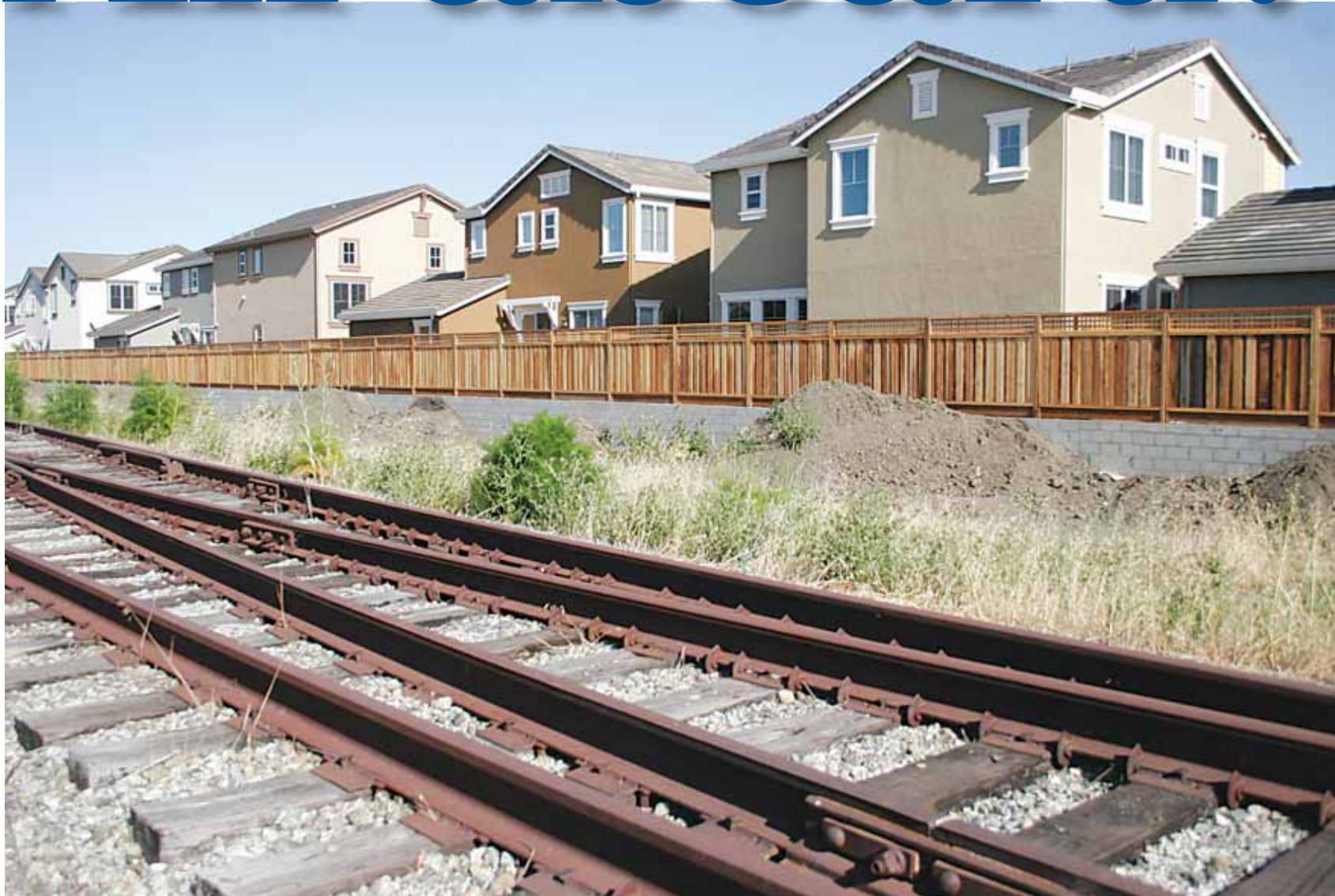
The Dumbarton rail line in Redwood City, but plans are moving forward connecting Menlo Park and Redwood City.
