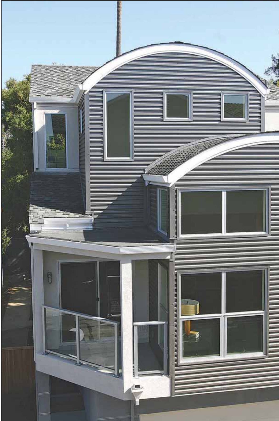
Clarum Homes bills its new 12-house development at 996 Willow in Menlo Park as energy-efficient 'Enviro-homes,' with energy consumption reduced by up to 90 percent.
