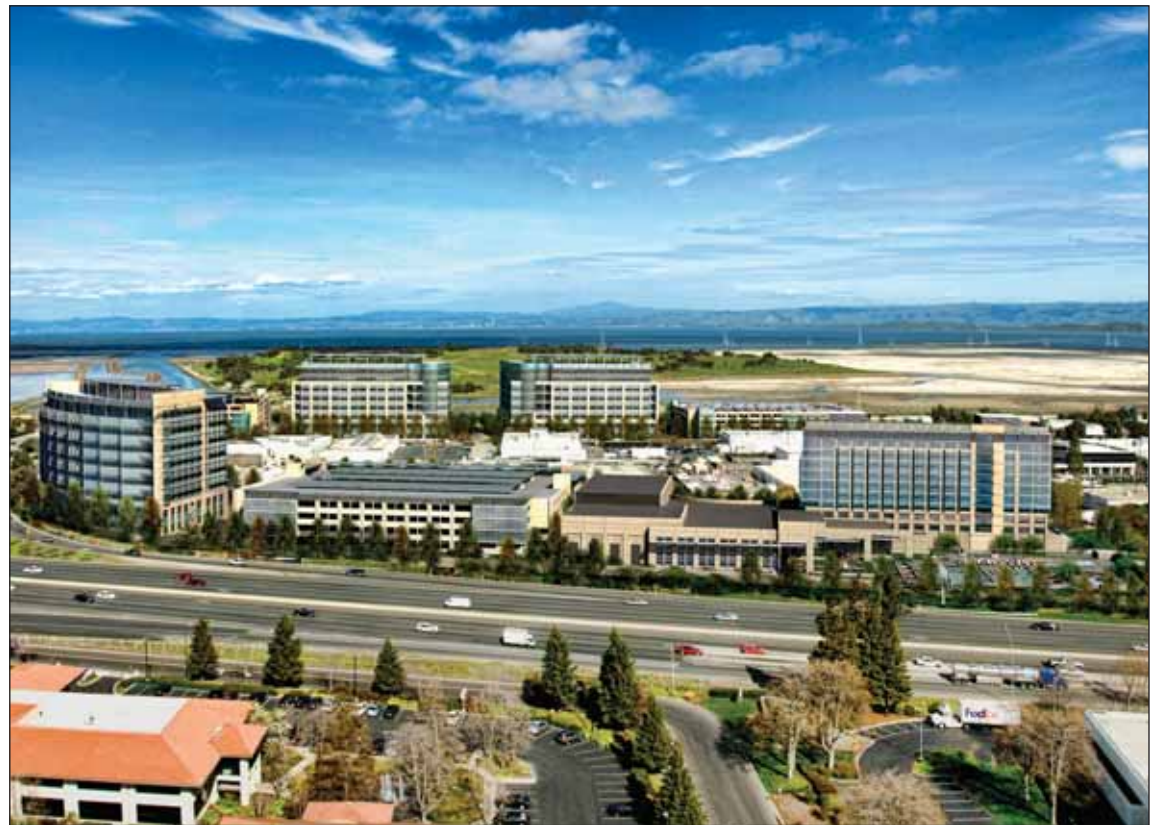
Looking across U.S. 101 toward Bedwell-Bayfront Park at the Menlo Gateway project proposed by developer David Bohannon. The project would consist of three eight-story office buildings, a 230-room hotel, a fitness center, and several parking garages. Rendering by DES Architects.
