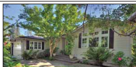
MENLO PARK $2,295,000 This one-level 4bd/3.5ba home, located in desirable Felton Gables, is on a .25+/- acre lot. This home was completely remodeled and expanded in 2006.
