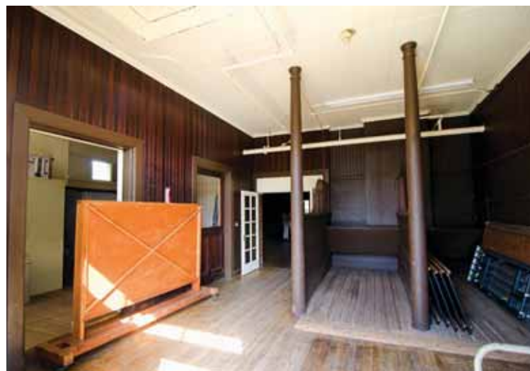
The stable room has two horse stalls, right.
