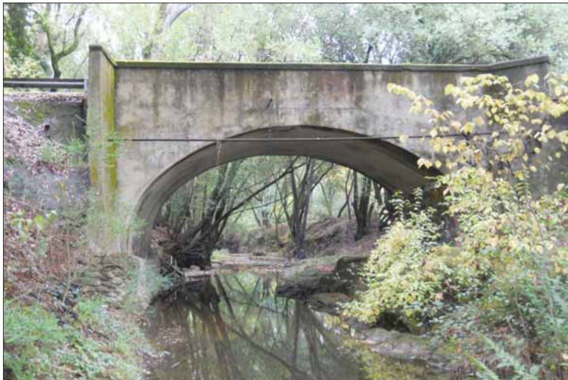
Photo by Quincy Engineering
