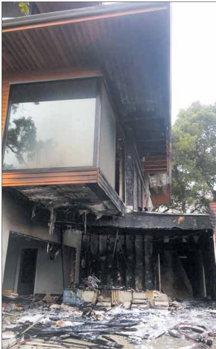
Photo by Rob Lindner, Woodside Fire Protection District
