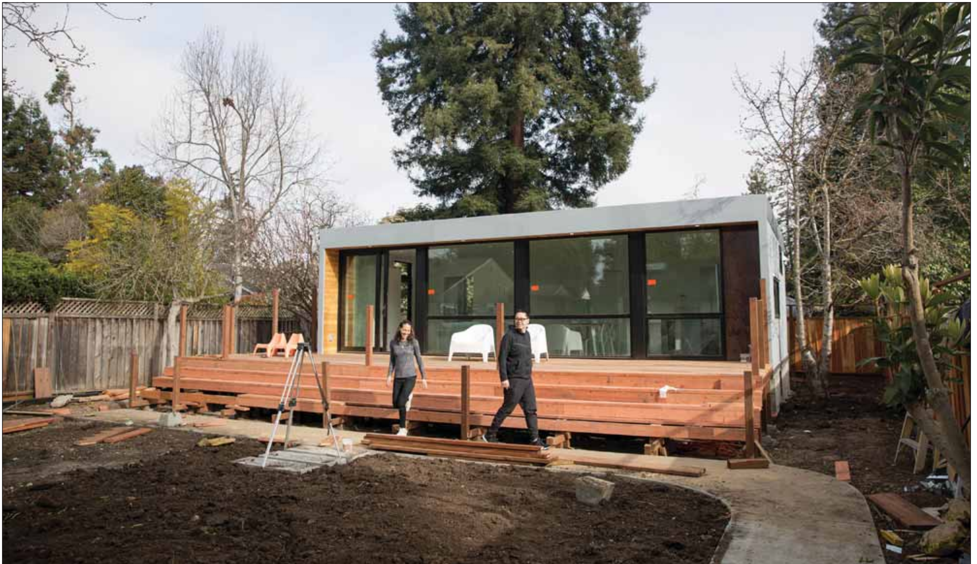
The To family's nonprofit, Soup, has hired an executive director to help other Bay Area homeowners build backyard houses and rent them to low-income tenants.
