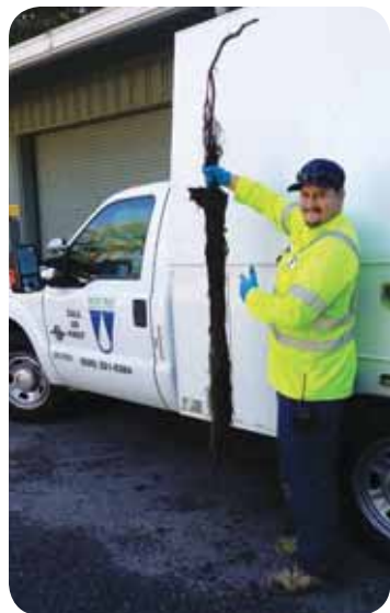
Roots, such as this one displayed by Justin Kinder, are a common cause of sewer damage.
