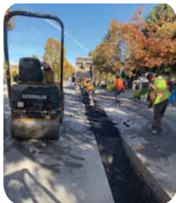
Over two miles of pipe is being replaced in the Belle Haven area.
