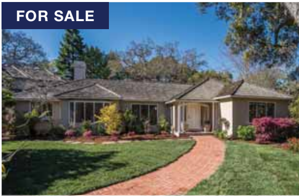
Stylish Remodel in Lindenwood
