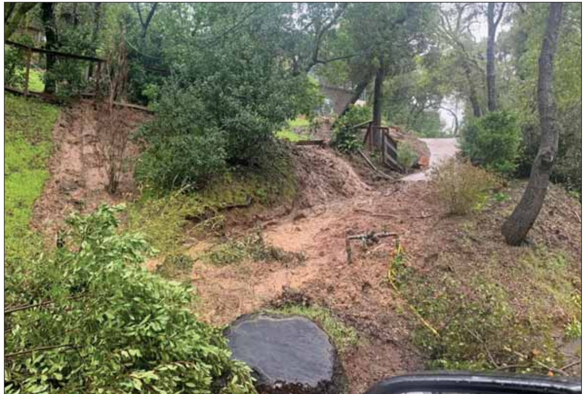
A mudslide off Patrol Road in Woodside on March 22.
