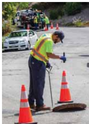
Inspecting Manhole Pipeline Access while Jetting
