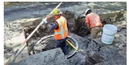
Contractor Replacing Old Brick Manhole with Concrete Manhole
