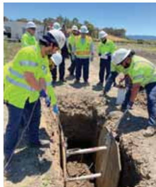
Trench Safety Training
