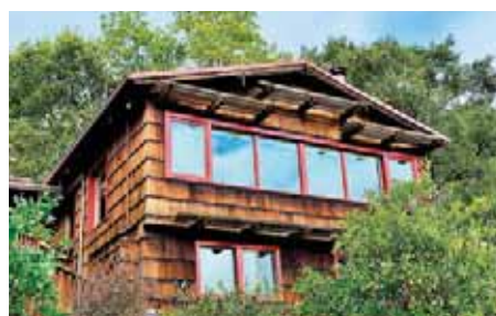
108 Santa Maria Avenue, Portola Valley
