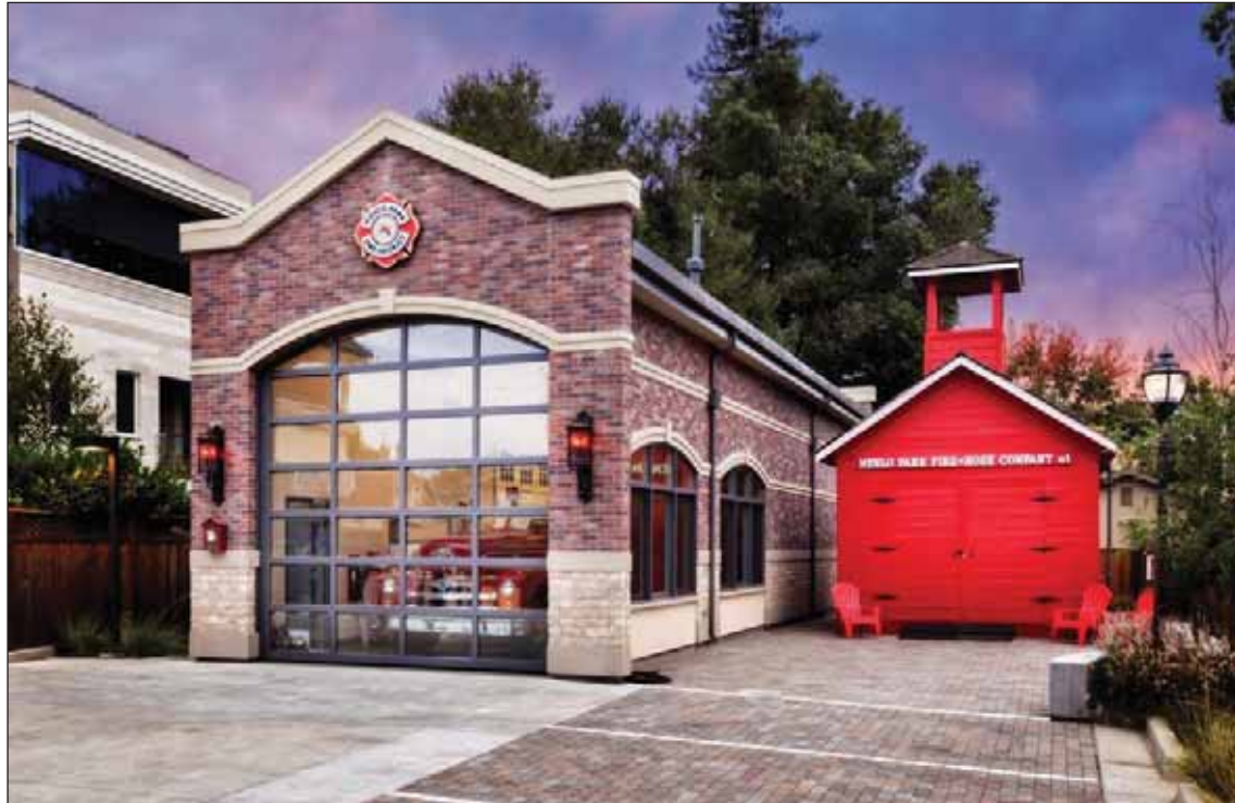
Courtesy Menlo Park Fire Protection District
